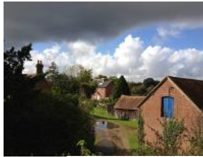
Photographs of a recently completed rural affordable housing scheme in Breamore, New Forest
