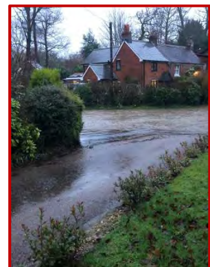
Flooding in the Old Romsey Road/Cadnam Lane area of Cadnam, on Sunday 16 th January 2020
